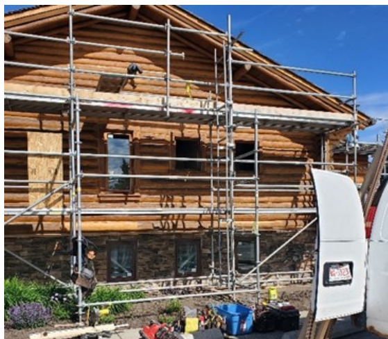
Scaffolding and window replacements on East wall
