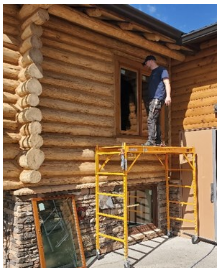
North wall of main room
