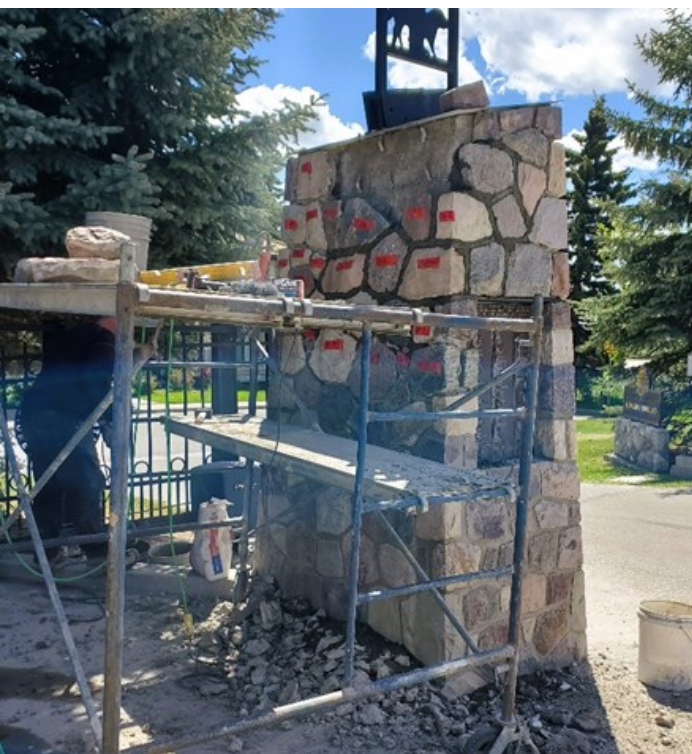
Front gate pedestal repairs
