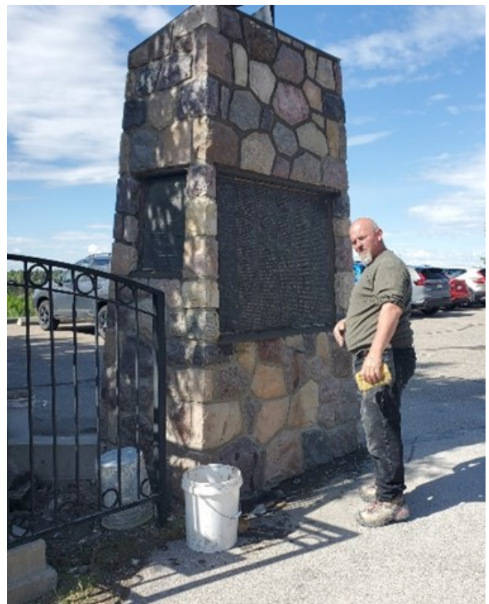
Stone Mason Martin puts finishing touches on the gate pedestal
