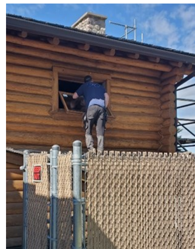
South facing Ladies Room
