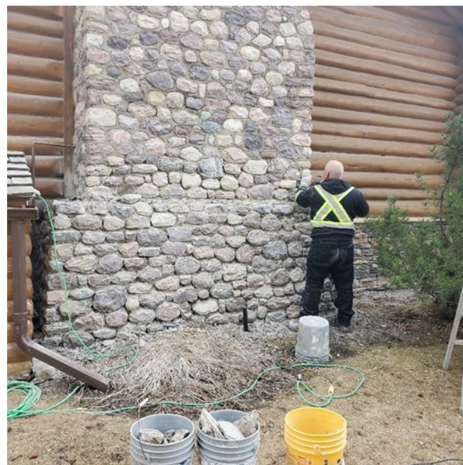
Stone Mason Martin working on the chimney
