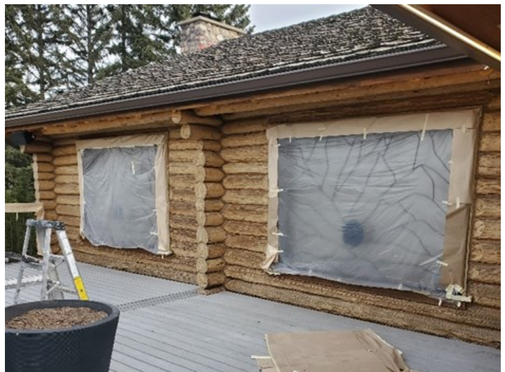
Logs stripped on deck
