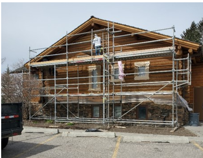
Painter stripping logs on the East Wall
