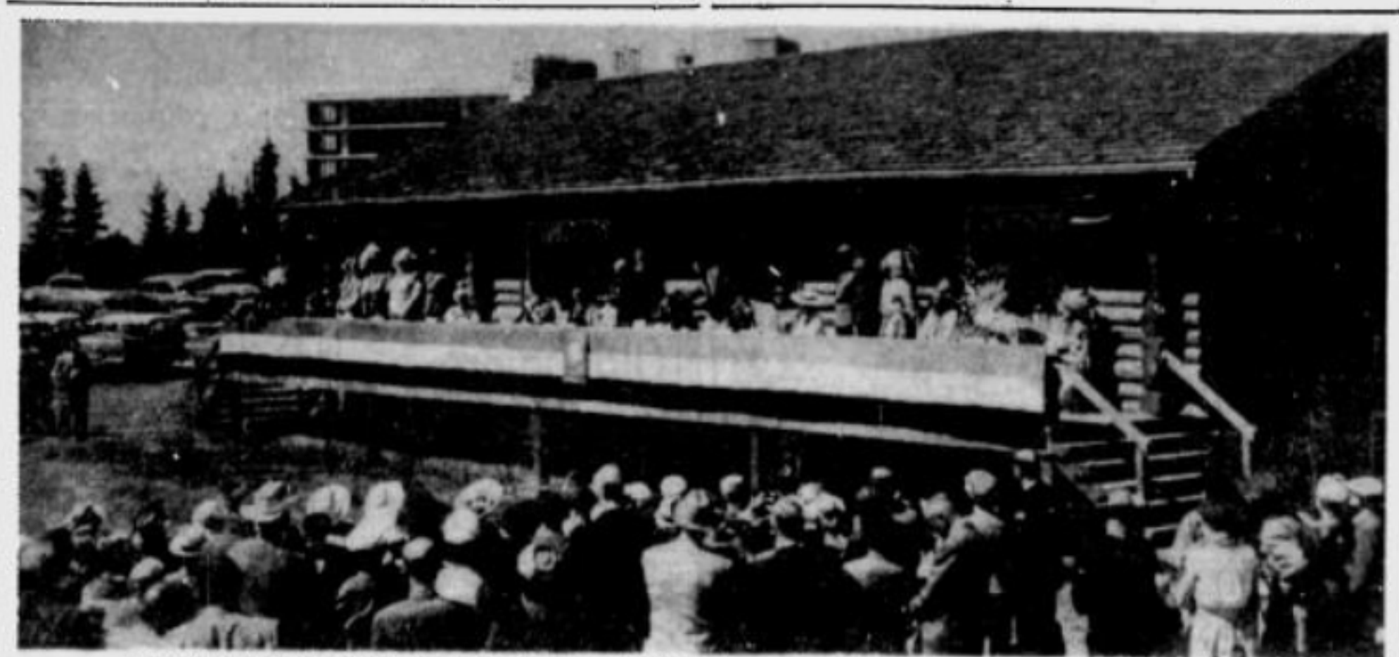
THE $50,000 PIONEER MEMORIAL BUILDING above the Elbow River was officially opened Wednesday by His Honor J. J. Bowlen, Lieutenant-Governor of Alberta. The top photo shows the exterior of the building, while the lower photo shows the interior looking toward the front door.
